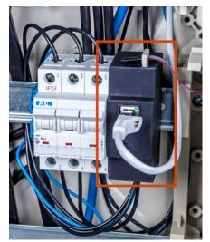
Figure 3 Three-sensor arrangement suitable for the monitoring of an induction motor
