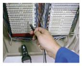
This locating method requires the use of a test tip which is part of a standard set.
